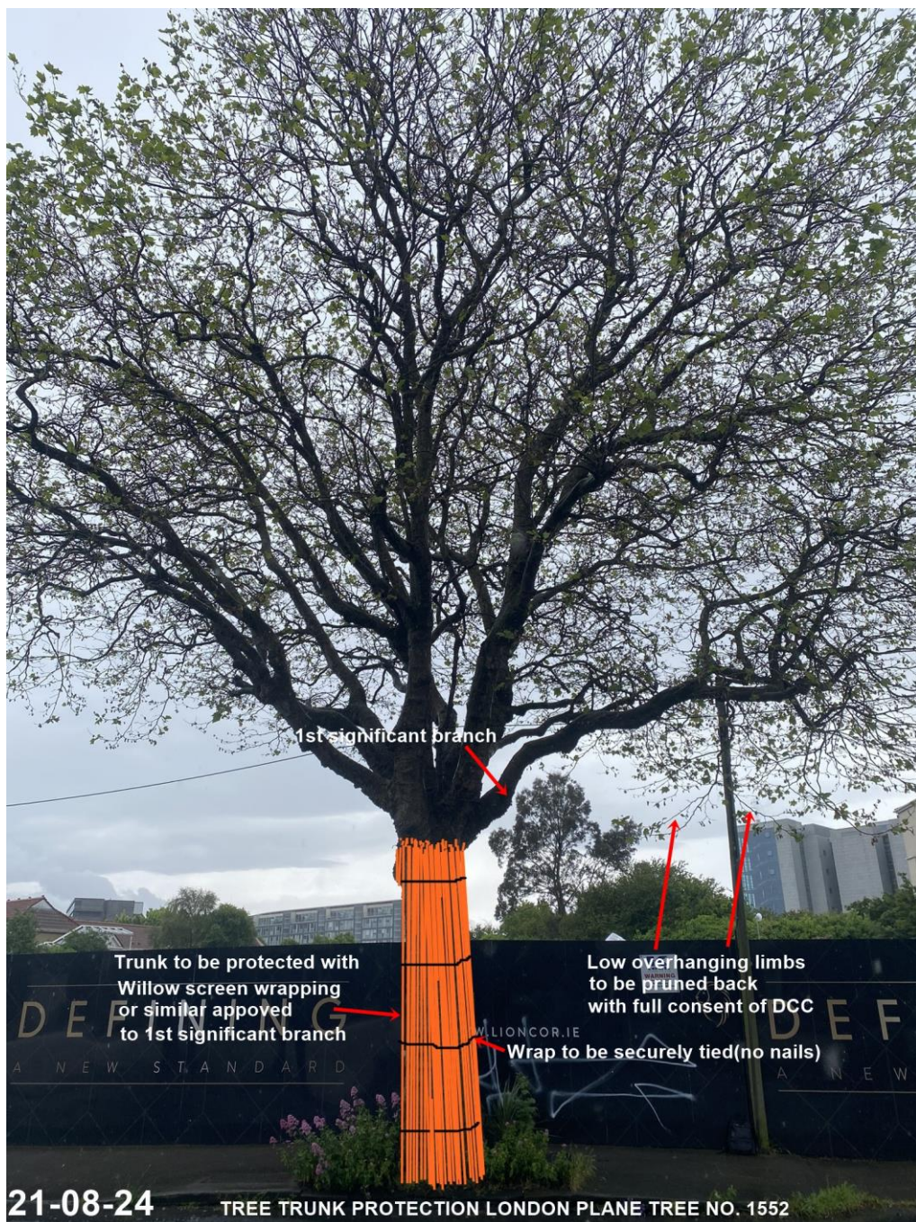
Image 2. Example of Tree Trunk Protection with Willow screen wrapping (or similar approved).
