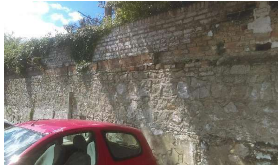
Plate 6: Western wall showing brick upper portion, facing southwest
