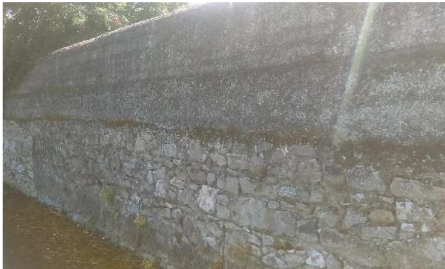
Plate 7: Wall at the southern limit of the site, facing east
