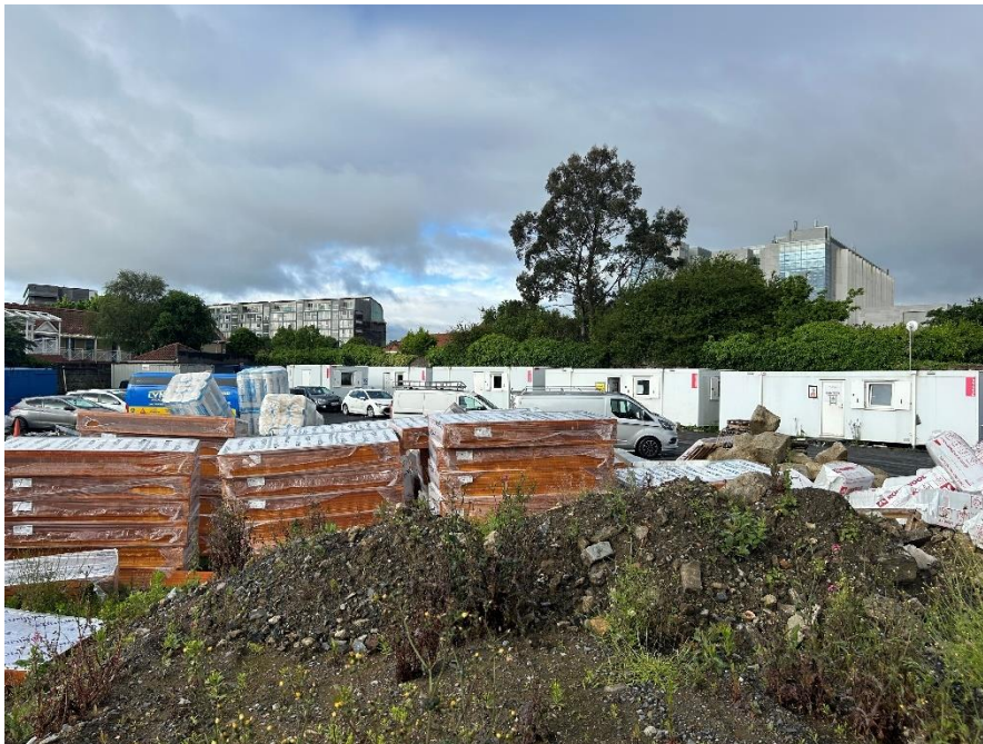
Plate 20 View of temporary structures to west of site
