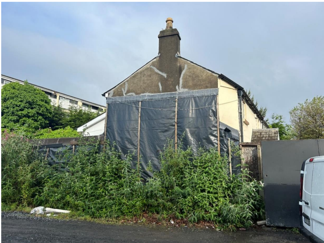
Plate 10 Shared boundary with No.167 Merrion Road
