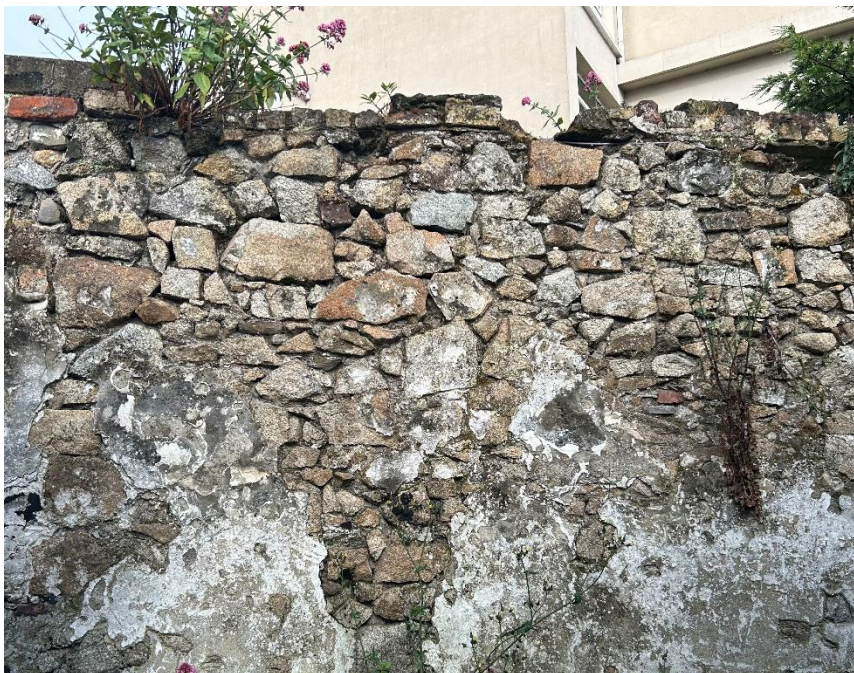
Plate 2 Walled boundary to the west, with intact fragments of plaster
