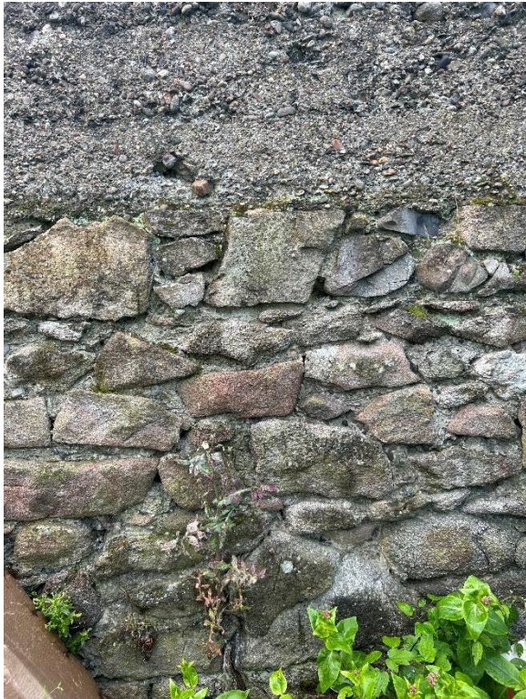
Plate 18 Detail of concrete capping above original rubble section
